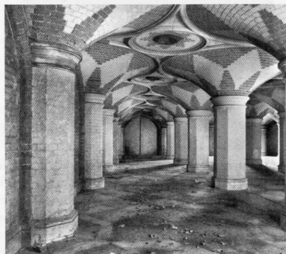
Crystal Palace High Level Subway. Photo by Nick Catford
